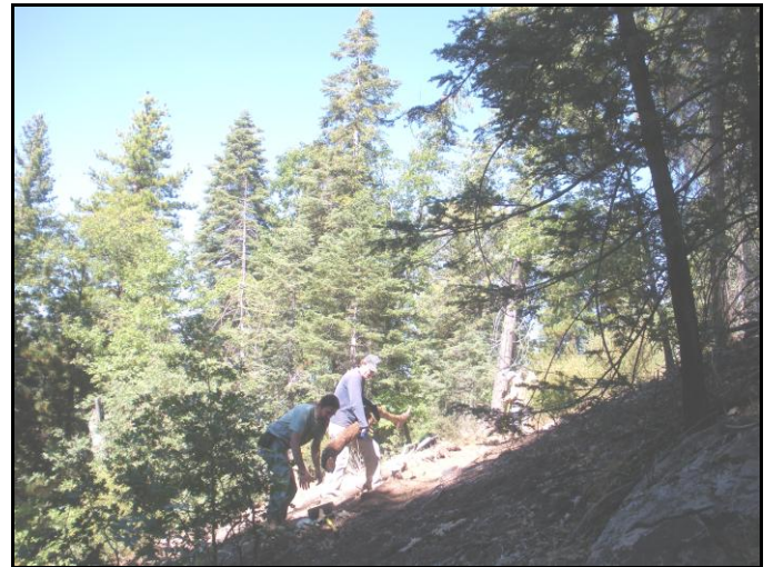
The "Trail Crew" hard at work on the Eagle Ridge trail.
